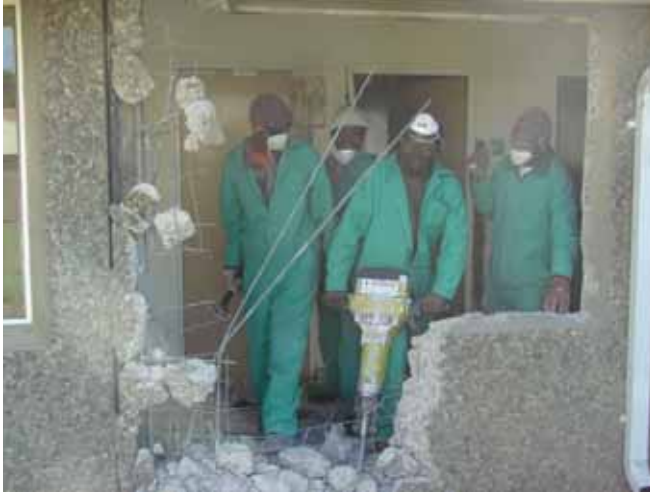
Figure 5.1 Newtown ablution upgrading.
